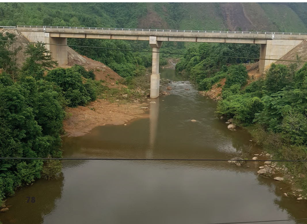
Fig. 81 | Cu De River with the new highway construction. 2019. (own)
