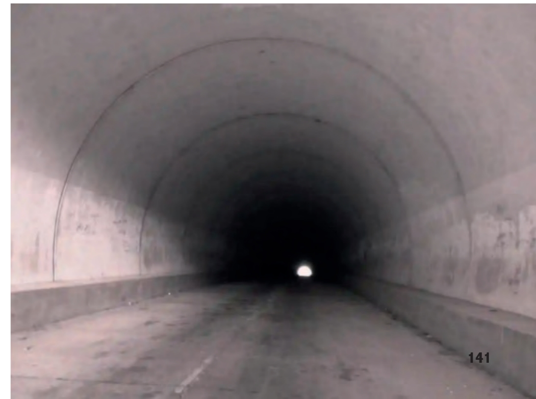
Fig. 169 | Tunnel along Ho-Chi-Minh Road. 2019. (own)
