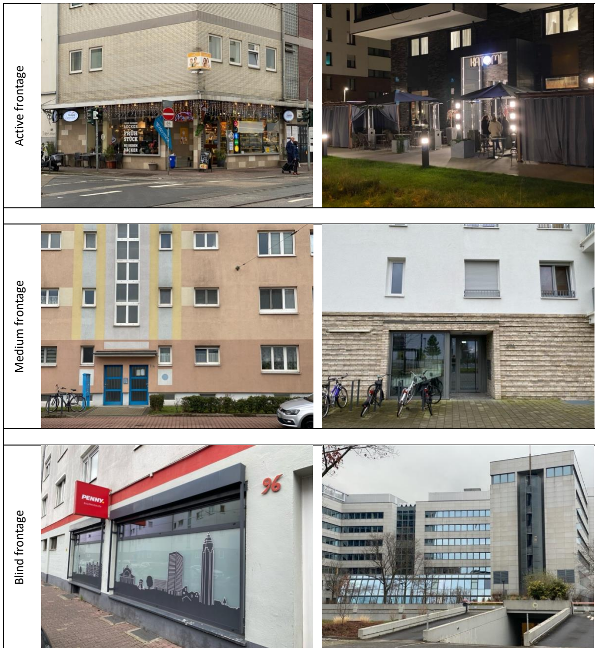
Figure 36. A visual comparison of active, medium, and blind building frontage in Niederrad Source: Author
