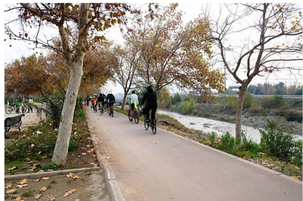
Figure 54. Section of the new cycle routes along the Mapocho river linear park. Source: Santiago mobility plan (STGO, 2019).
