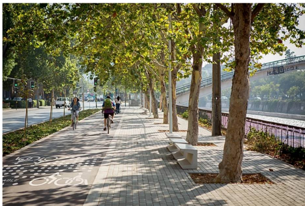
Figure 53. Section of the new cycle routes along one of the streets of the CicloRecreovia network. Source: Santiago mobility plan (STGO, 2019).
