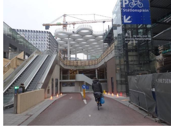
Figure 28. Utrecht Centraal bike parking ride-in access. Source: archdaily.com (2021).
